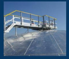
TORAY PLASTICS AN3 STORAGE TANK, PRAI Completed in 2014, this dome roof tank with 19.5m diameter x 20m height, total tonnage of 146 MT, was built in a live plant with limited space. We had devised a new construction technique and incorporated automatic welding processes that enabled us to complete the construction within record time.
