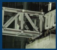
GUIDEWAY STEEL STRUCTURE, SUBANG JAYA Spanning 55m in length and 9m in width, the 280 MT guideway was fully constructed in our factory in 5 segments and delivered to site for installation. Splice joints at the ends of each segment were fabricated with laser precision joint alignment.
