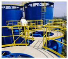
Based in Tuas, Singapore, this project consists of 6 base oil storage tanks, 3 blending tanks, and an additive tank with 50mm insulation. The base oil tanks were constructed at the Tuas site, and the remaining four smaller tanks were transported in two assemblies for site assembly and installation. Total tonnage was 250 MT, completed in 2018.
