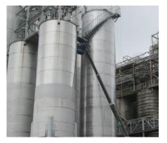
Completed in 2014, this silo for storing pellet with a dimension of Ø4500 x 25,000mmH (25 MT) was built completely in our plant. The silo was then transported wholly to site and installed with a single lift. Site installation activity was completed within a day, together with connecting spiral staircase which was delivered as a separate package.
